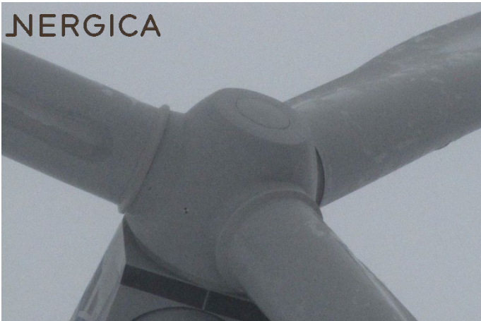
Figure 7: Typical glaze accumulation on wind turbine rotor
