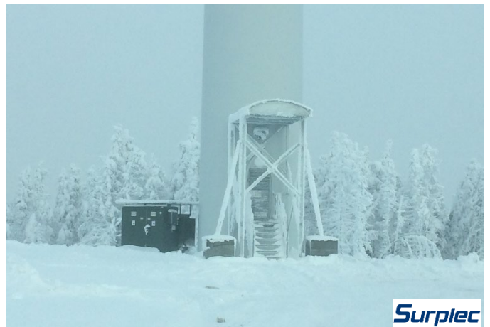
Figure 14: Permanent ice protection device for tower entrance
