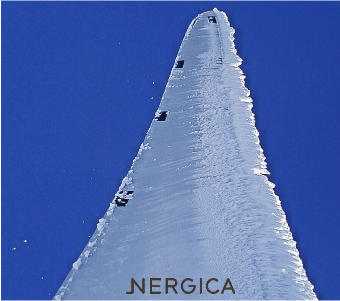
Figure 6: Heavy rime on a wind turbine blade
