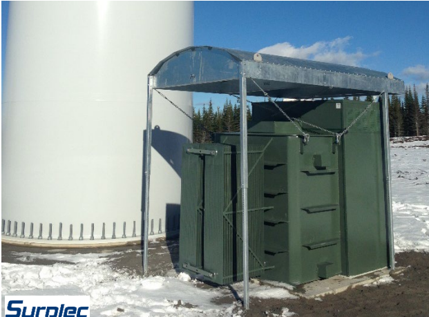
Figure 15: Permanent ice protection device for transformers
