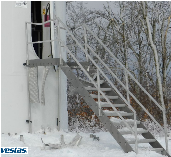
Figure 19: Damaged stairs from an ice fall
