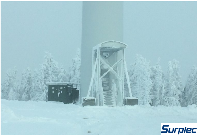
Figure 14: Permanent ice protection device for tower entrance
