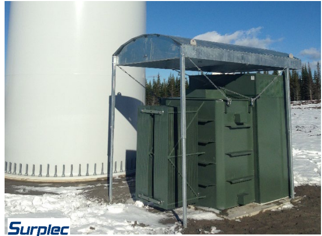
Figure 15: Permanent ice protection device for transformers
