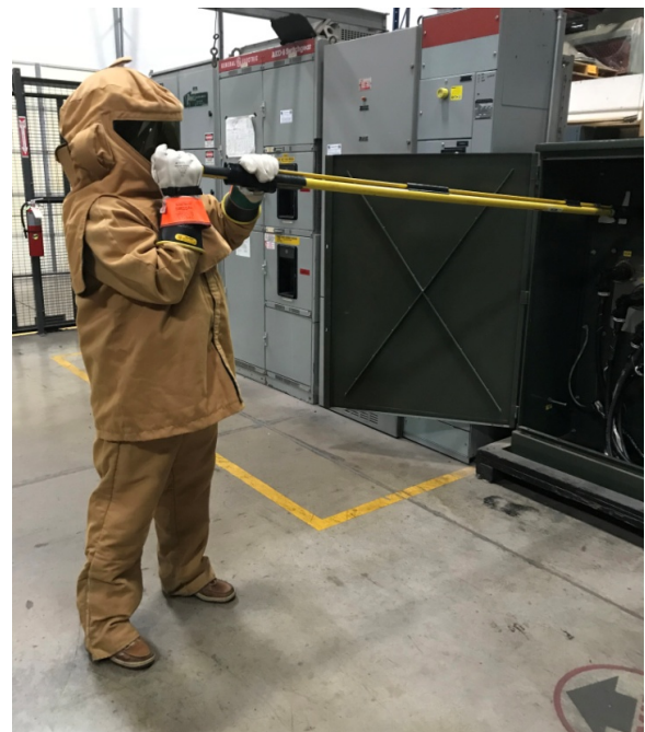
The photo above, taken at a training facility, shows the proper PPE and live-line tool to be used for operating the bypass switch.
