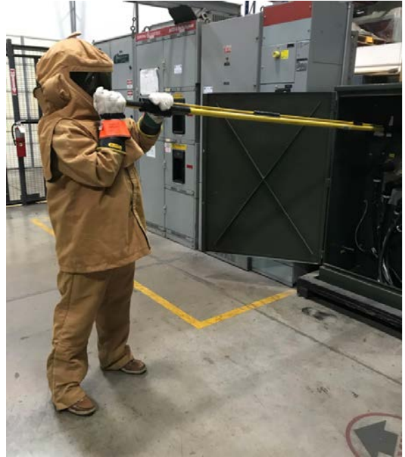
The photo above, taken at a training facility, shows the proper PPE and live-line tool to be used for operating the bypass switch.
